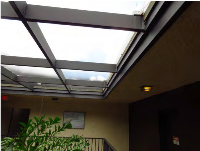
VIEW OF SKYLIGHT
