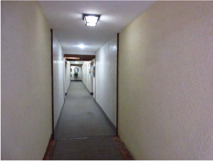
VIEW OF COMMON AREA HALLWAY
