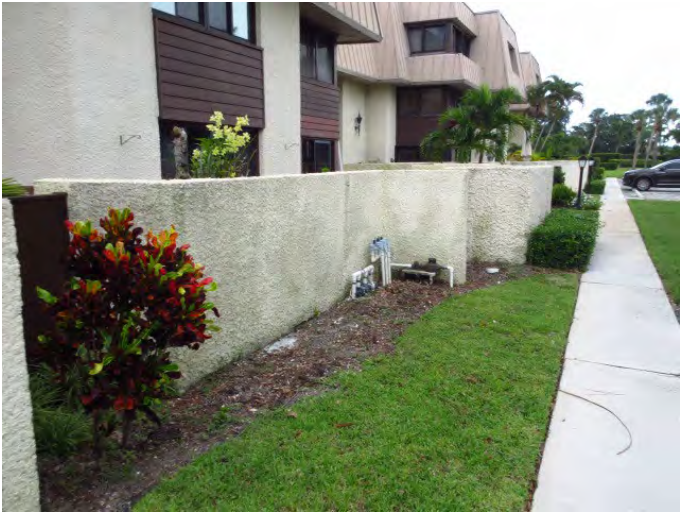
GENERAL VIEW OF LANDSCAPING AND SIDEWALK
