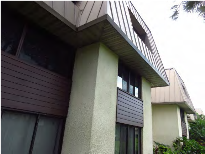
GENERAL VIEW OF BUILDING EXTERIOR FINISHES
