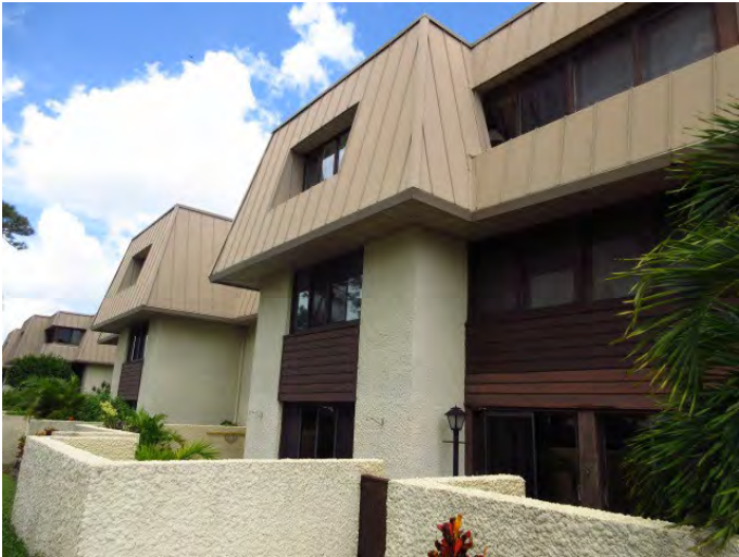
GENERAL VIEW OF BUILDING EXTERIOR FINISHES
