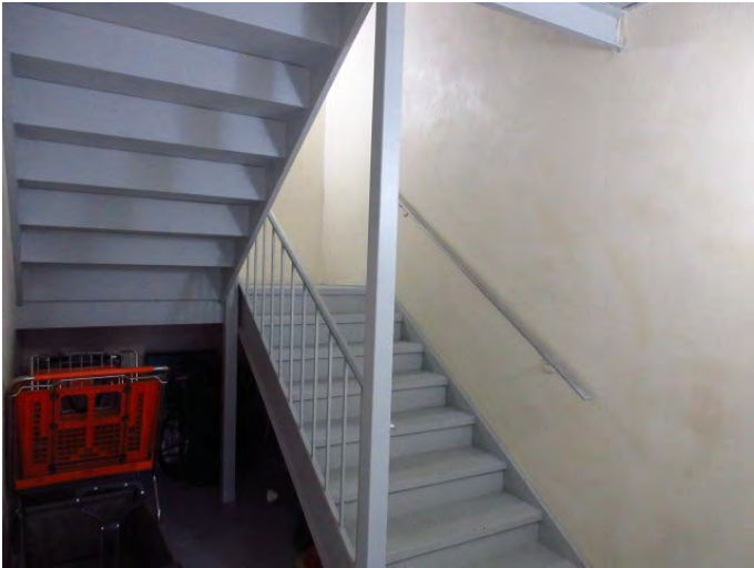
GENERAL VIEW OF INTERIOR STAIRS
