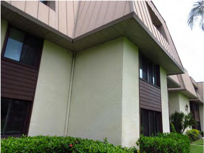
GENERAL VIEW OF BUILDING EXTERIOR FINISHES
