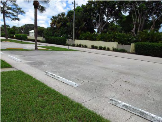
GENERAL VIEW OF PARKING AND PAVEMENT
