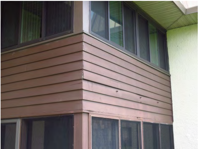
VIEW OF BUILDING EXTERIOR FINISHES
