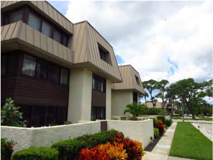
GENERAL VIEW OF BUILDING EXTERIOR FINISHES
