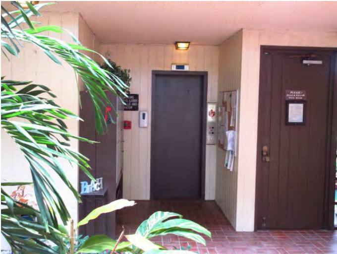
GENERAL VIEW OF ELEVATOR LOBBY
