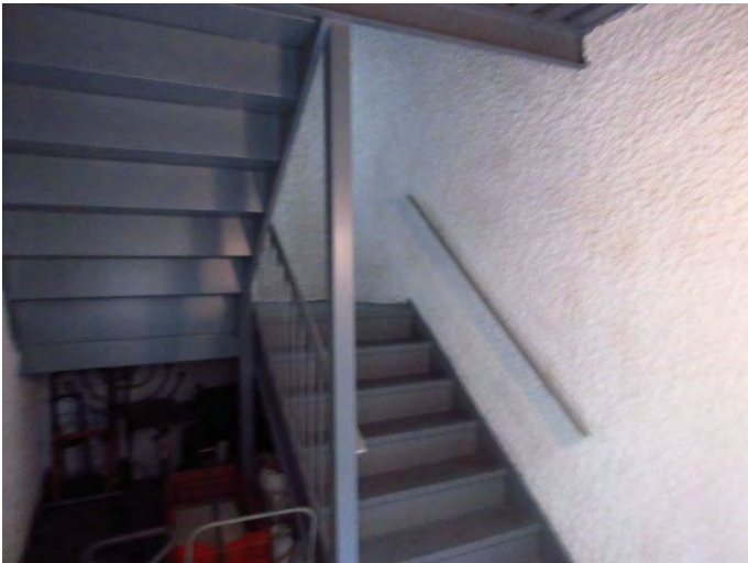
VIEW OF INTERIOR STAIRS
