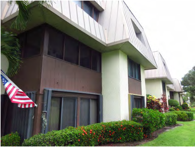
GENERAL VIEW OF BUILDING EXTERIOR FINISHES
