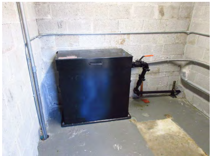
VIEW OF ELEVATOR EQUIPMENT
