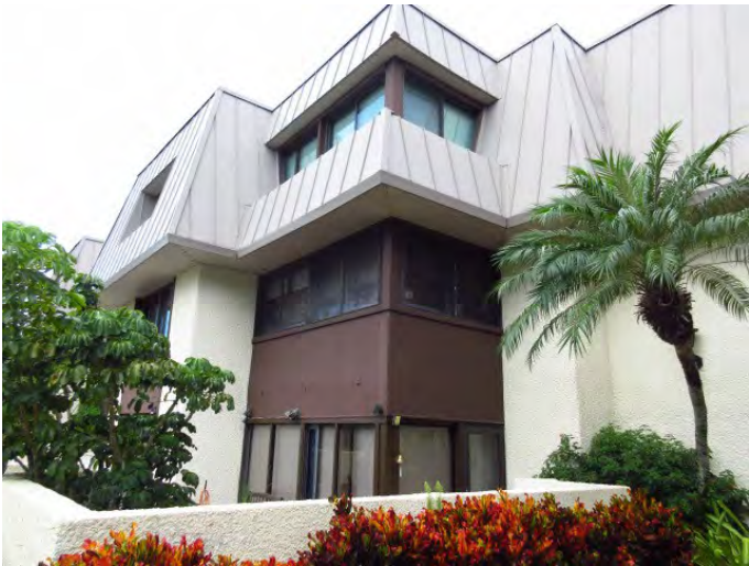
GENERAL VIEW OF BUILDING EXTERIOR FINISHES
