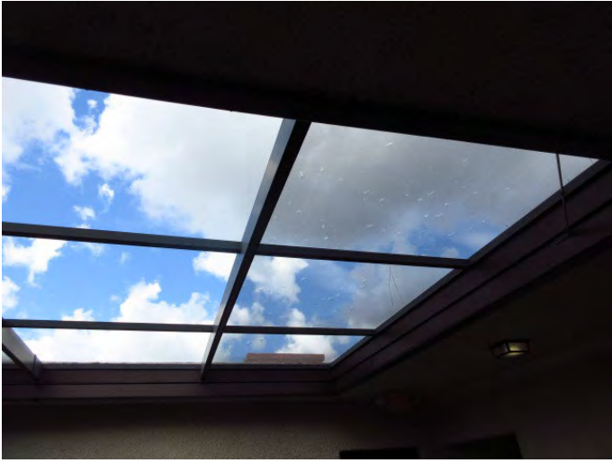
VIEW OF SKYLIGHT
