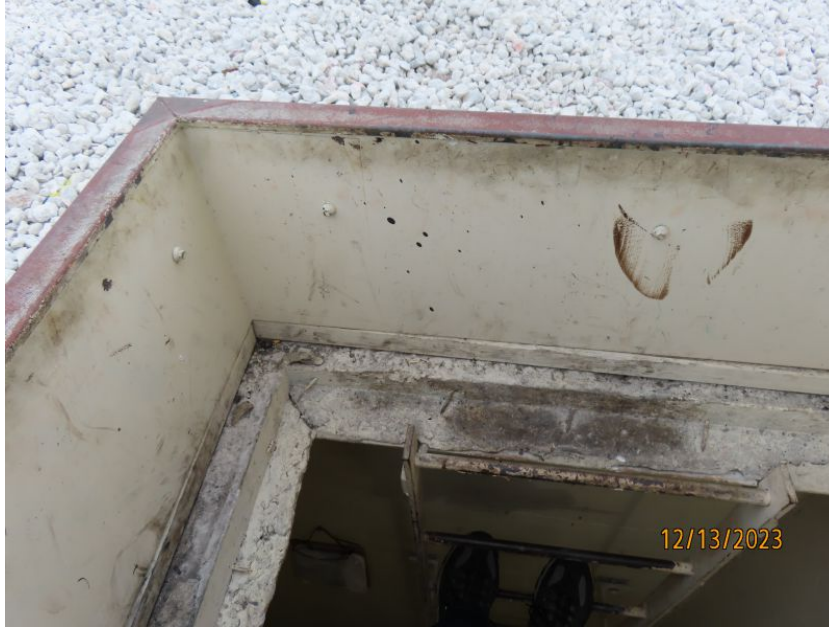
Reinforced Concrete Roof Deck
