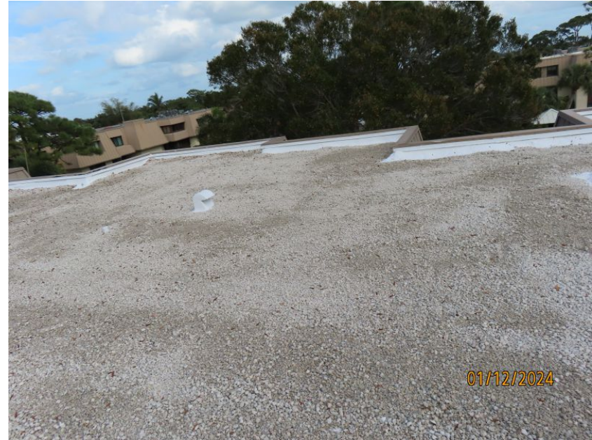
Built Up/Rolled Asphalt (Flat) Roof Covering
