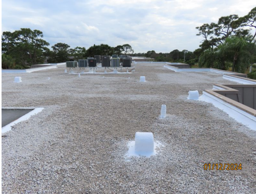
Built Up/Rolled Asphalt (Flat) Roof Covering
