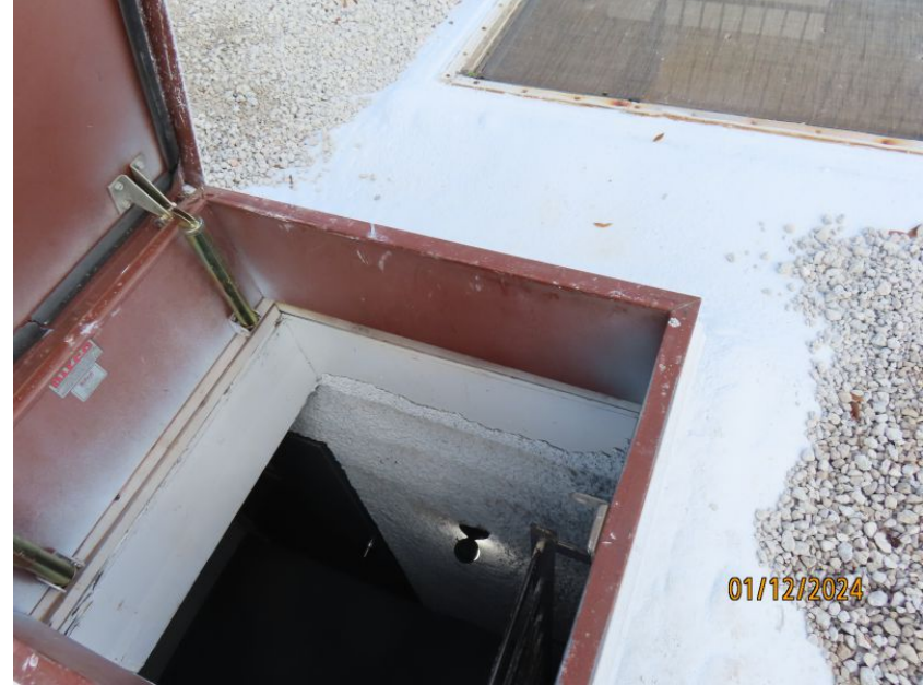
Reinforced Concrete Roof Deck
