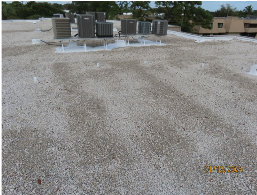
Built Up/Rolled Asphalt (Flat) Roof Covering
