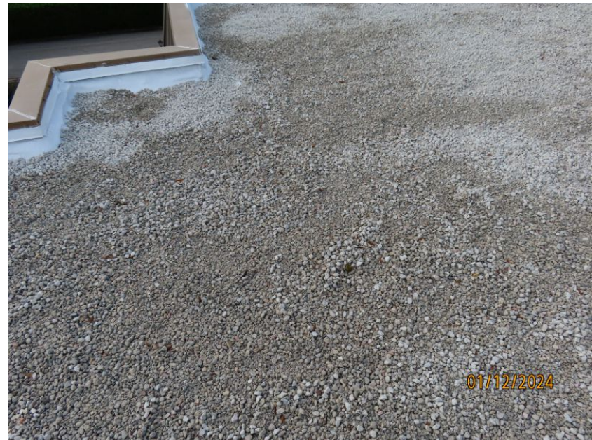
Built Up/Rolled Asphalt (Flat) Roof Covering
