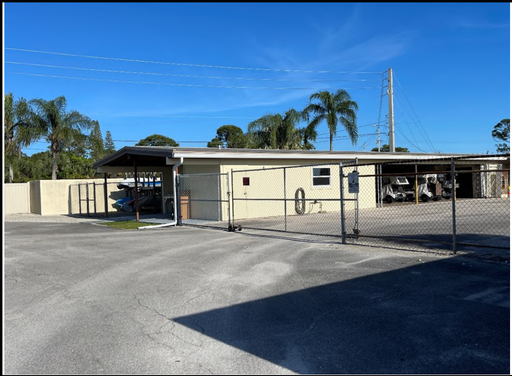
VIEW OF MAINTENANCE BUILDING
