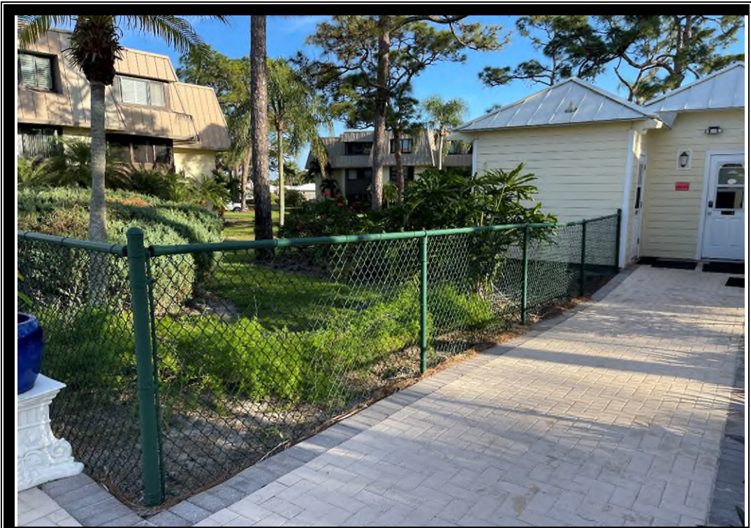
VIEW OF POOL FENCING
