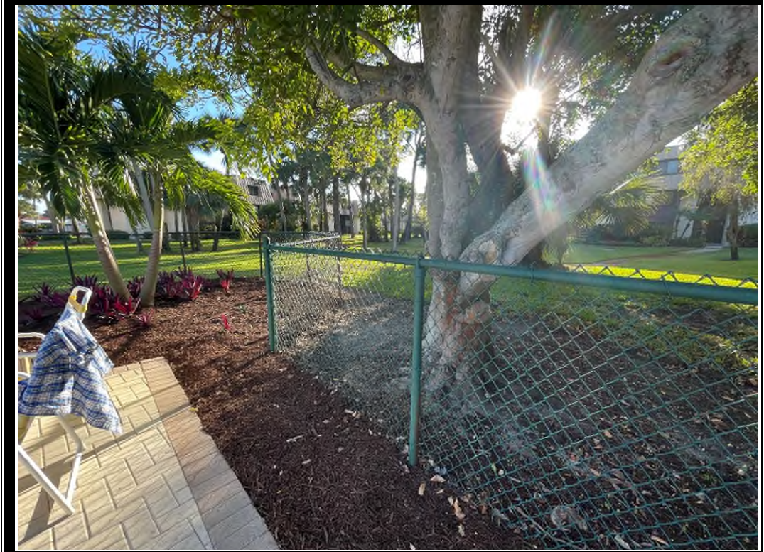
VIEW OF POOL FENCING
