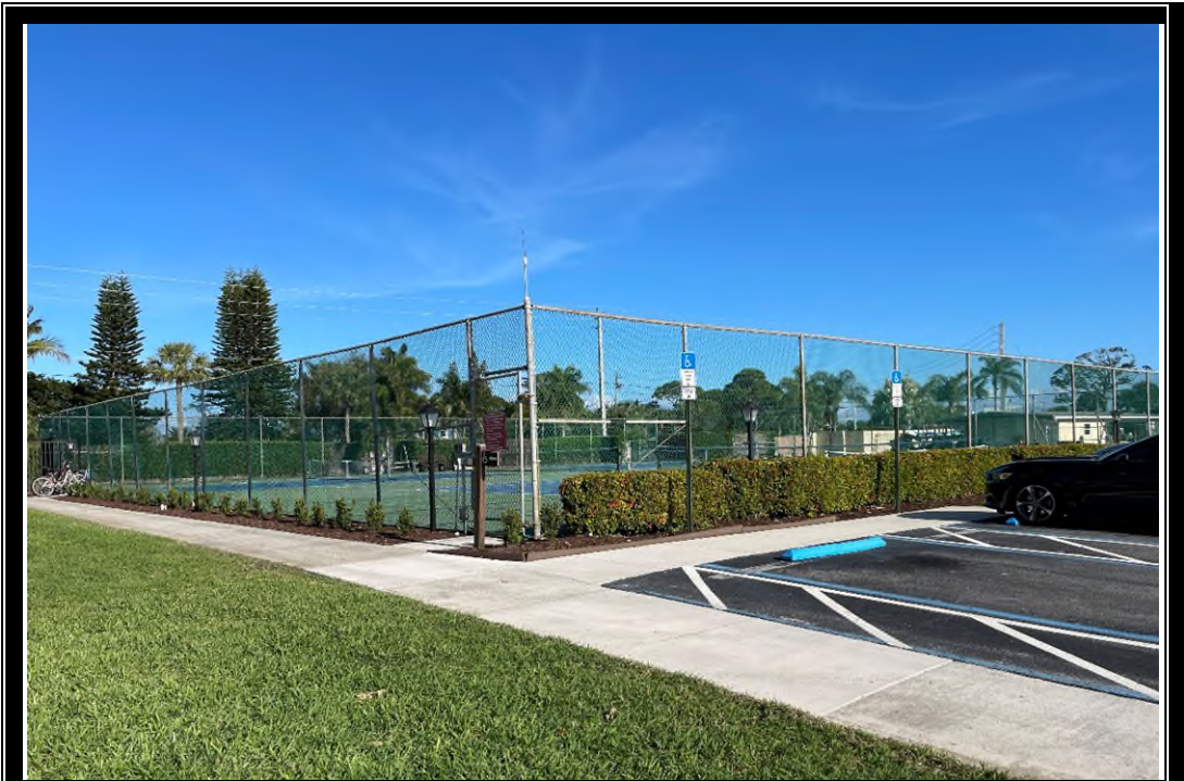
VIEW OF TENNIS COURTS AND FENCING
