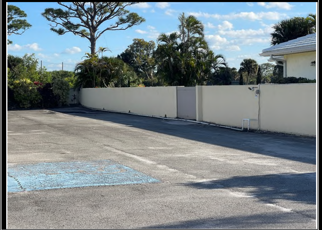
VIEW OF PERIMETER FENCING/WALL
