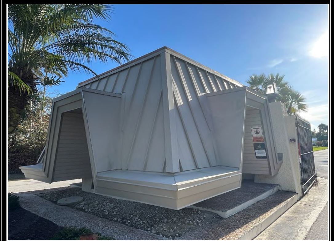
VIEW OF GUARD HOUSE
