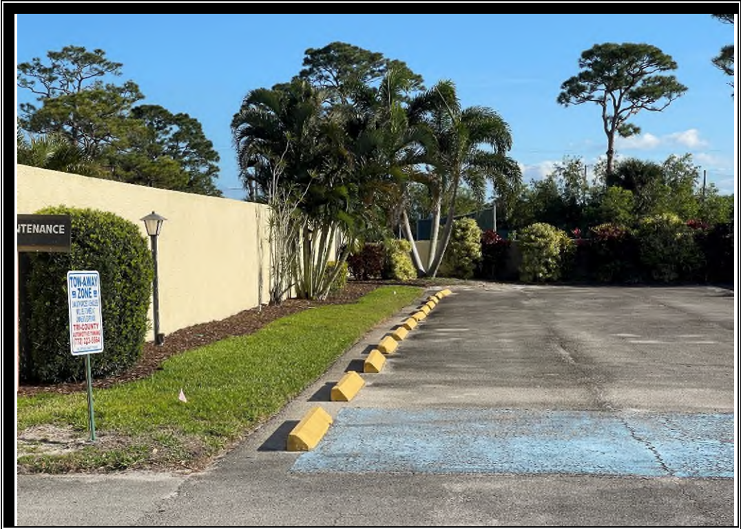
VIEW OF PERIMETER FENCING/WALL
