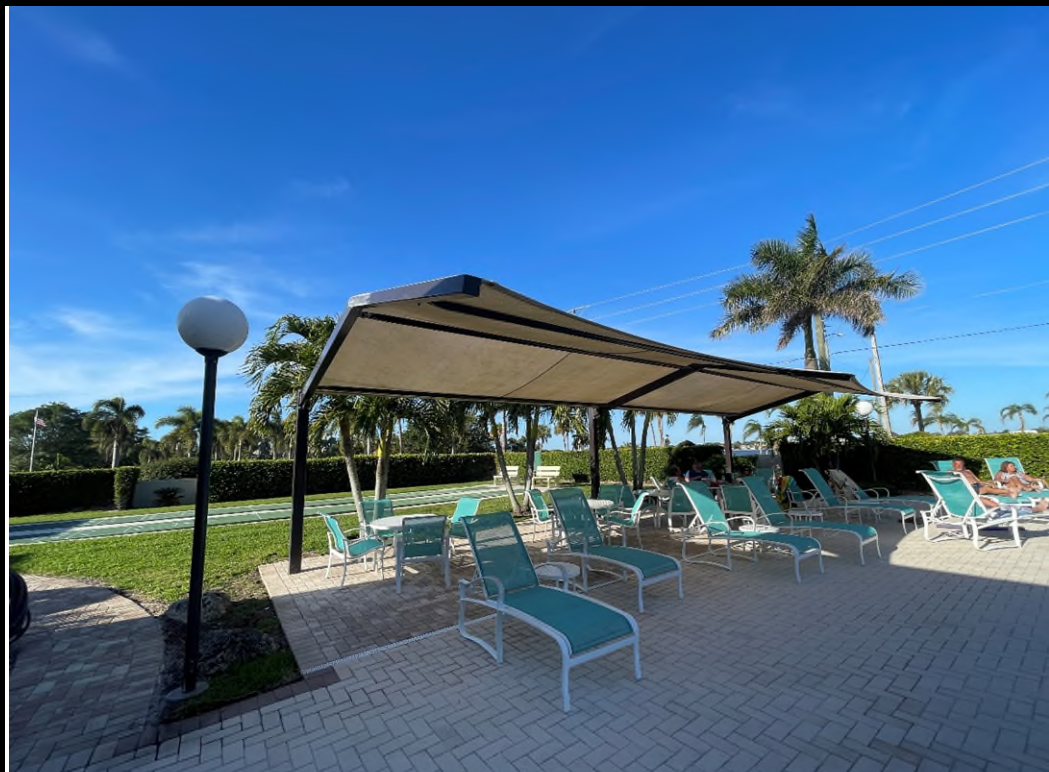
VIEW OF SHADE STRUCTURE
