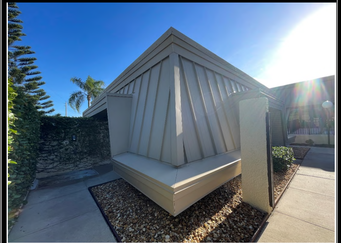
VIEW OF POOL HOUSE AT CLUBHOUSE
