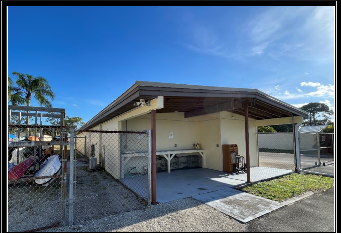
VIEW OF MAINTENANCE BUILDING
