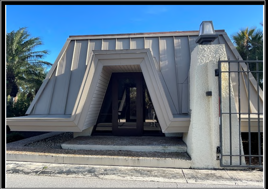
VIEW OF GUARD HOUSE
