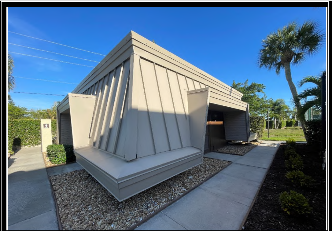
VIEW OF POOL HOUSE AT CLUBHOUSE
