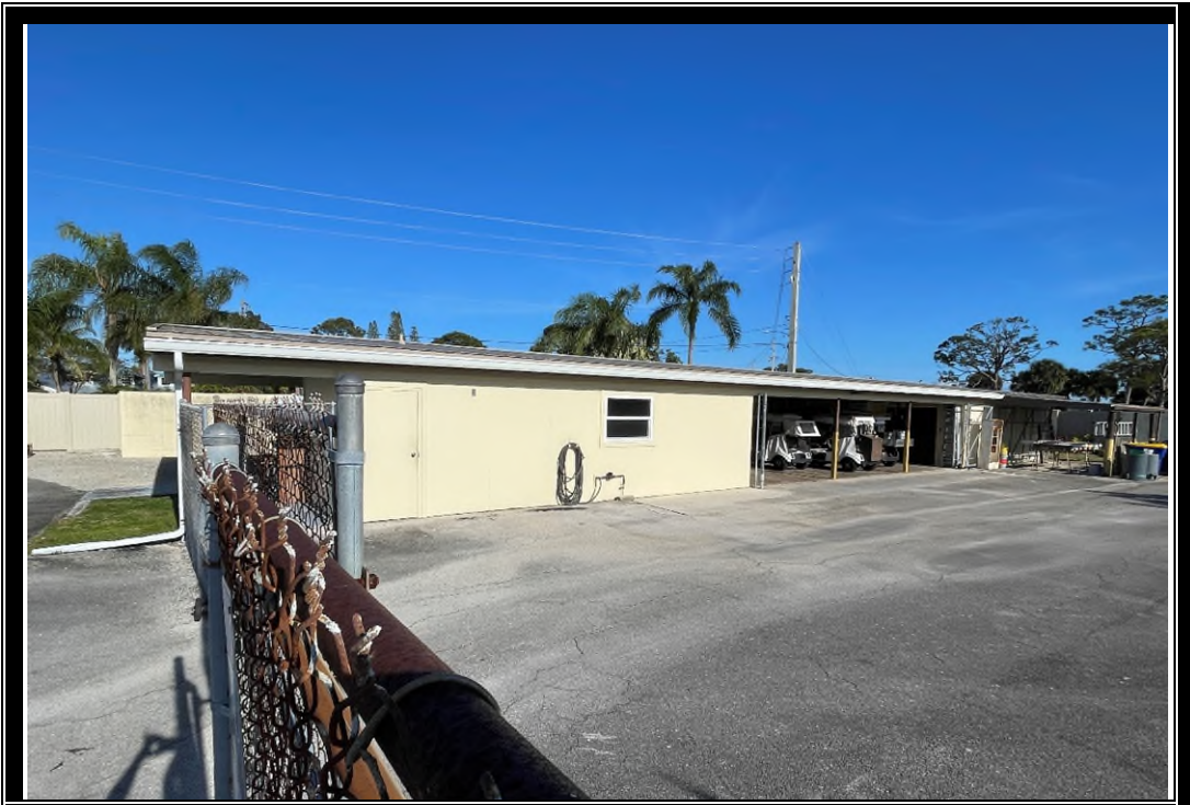
VIEW OF MAINTENANCE BUILDING
