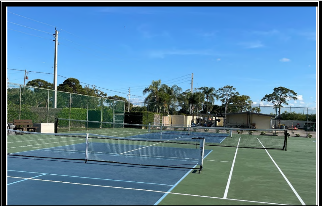
VIEW OF TENNIS COURTS AND FENCING
