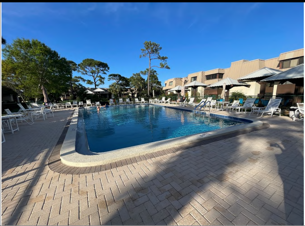
VIEW OF TYPICAL SWIMMING POOL # 2 & # 3
