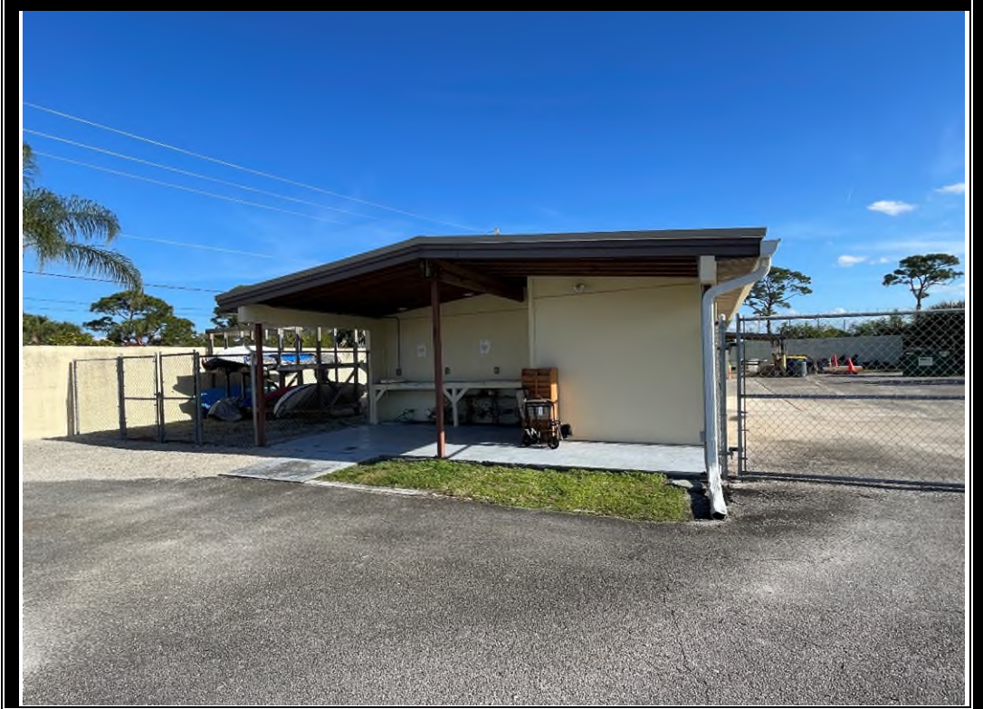
VIEW OF MAINTENANCE BUILDING
