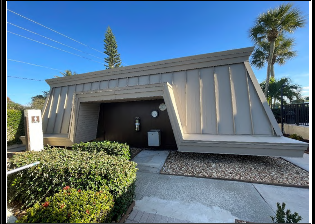
VIEW OF POOL HOUSE AT CLUBHOUSE
