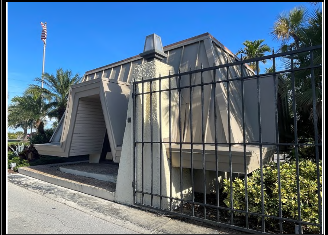
VIEW OF GUARD HOUSE
